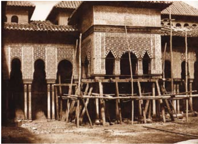
147. Gustave de Beaucorps, [ Oriental Temple of the Lion's Patio during Restoration Works ], ca. 1858. Ortiz Echagüe Legacy, University of Navarre, Spain.
