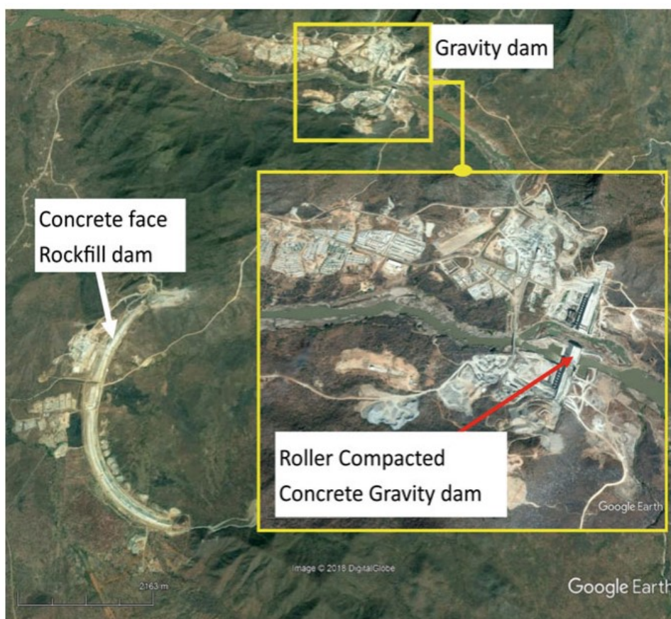
Fig. 2.2 Main RCC gravity dam and the supporting saddle dam (Source: Google earth, 2018).
