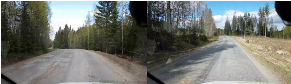
Figure 12. Person 1: severe hole. Computer vision: no hole identified (2 instances).
