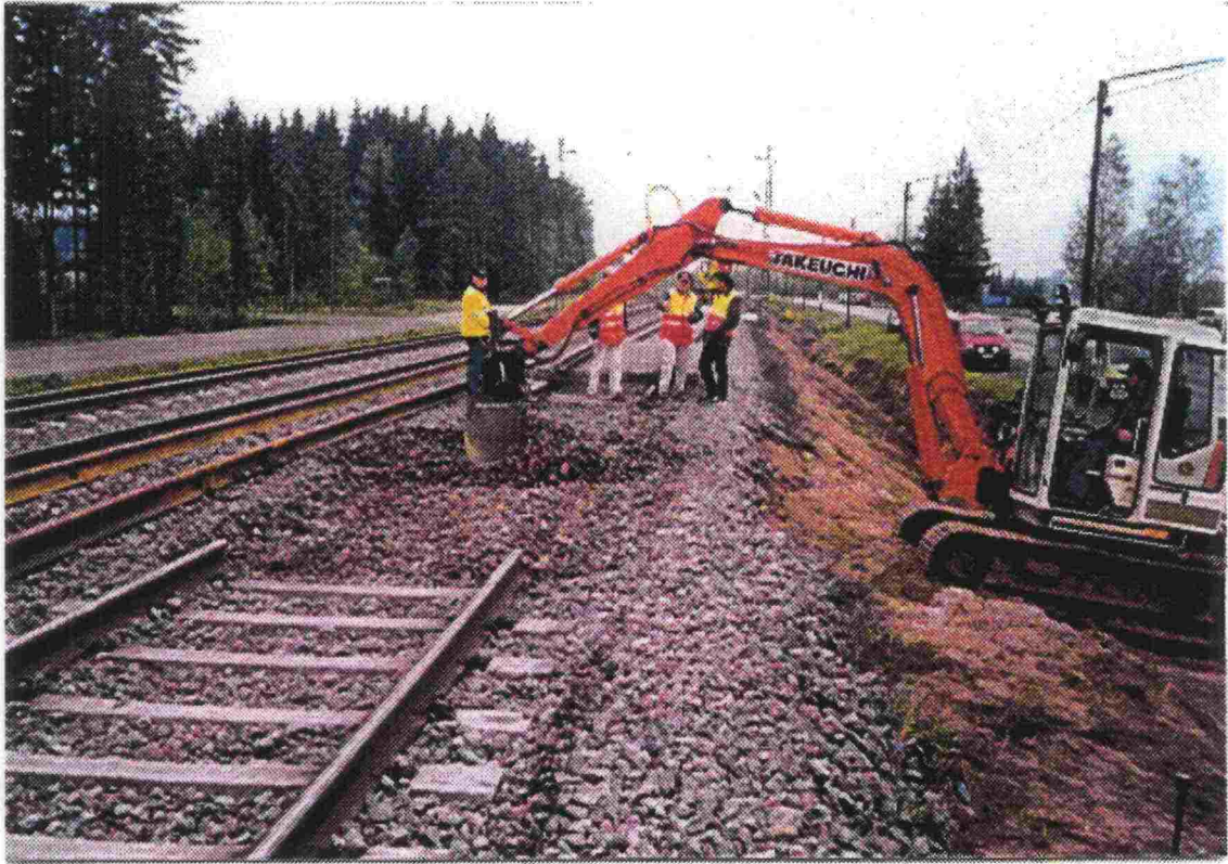
Figure 2.2:1 Cutting the track and excavating the embankment.
