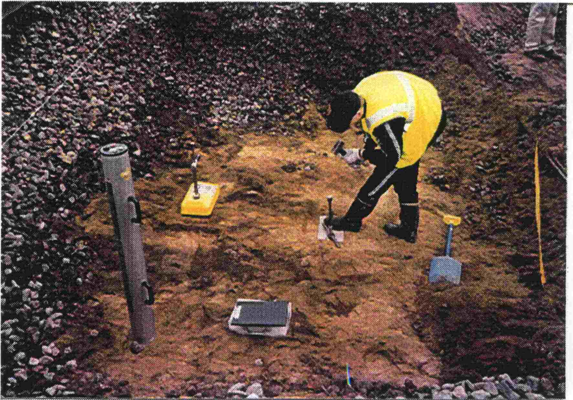
Figure 2.2:2 Measuring the density state of the embankment during the excavation.
