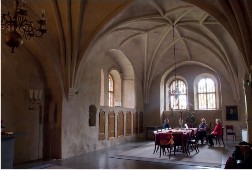
Fig. 5. The sacristy of Turku Cathedral. Part of the relic collection was found in a bricked-up recess in the wall in 1924. The recess, which now has a fitted wooden door, is the furthest one from the camera. Photo by Visa Immonen.
